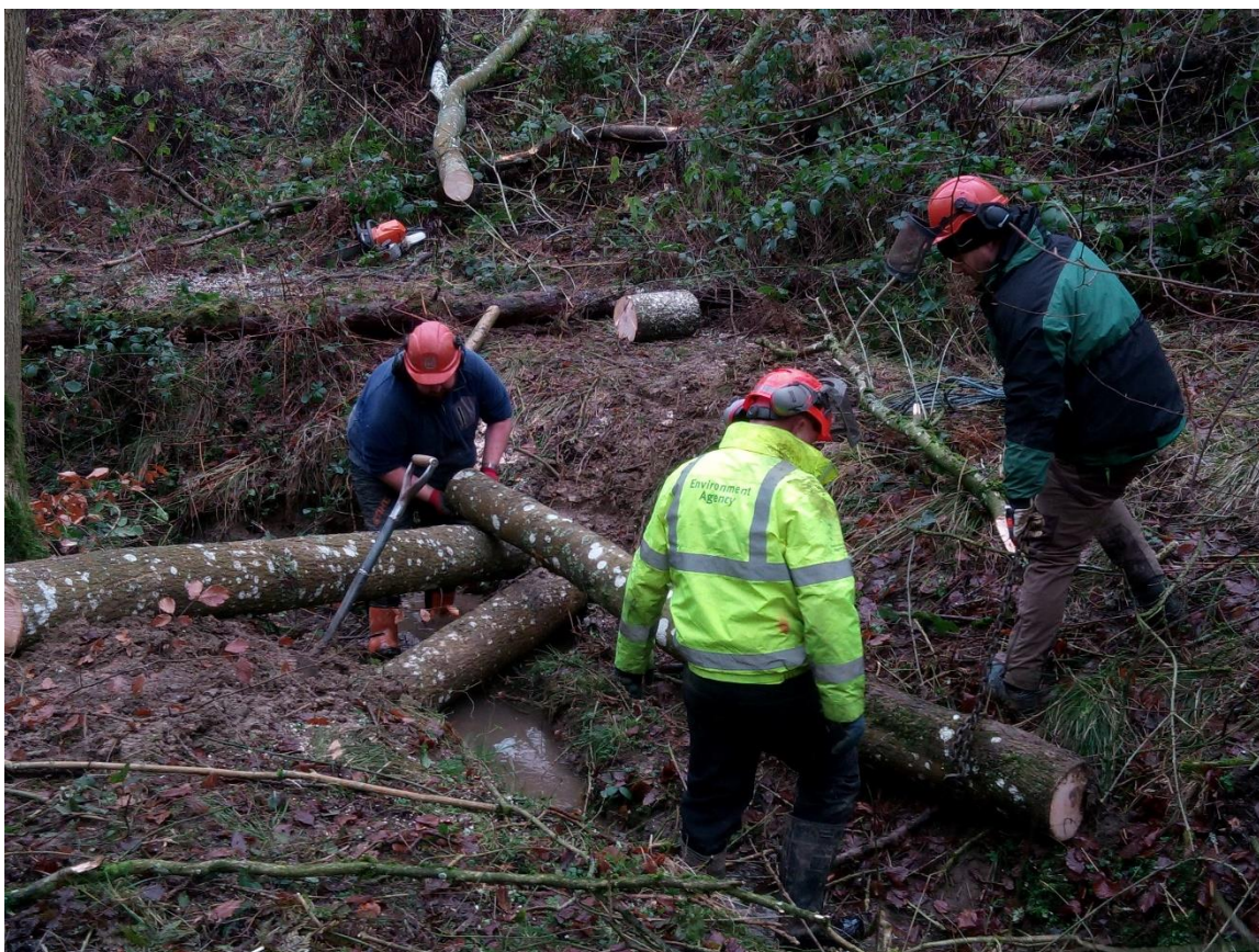
Figure 1 - Project partners working together to build leaky dams at Croft Castle
